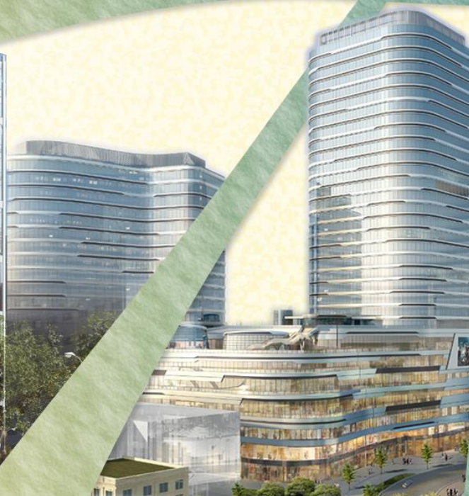
Haizhu Square Station Project, Guangzhou
