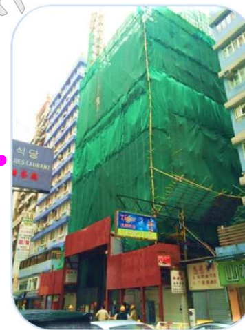
38-40A Hillwood Road in February 2016
