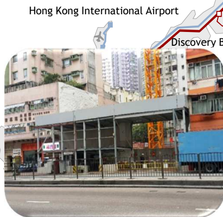
200 Ma Tau Wai Road project in March 2015
