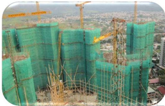
THE REACH - Tai Tong Road project in early Aug 2012
