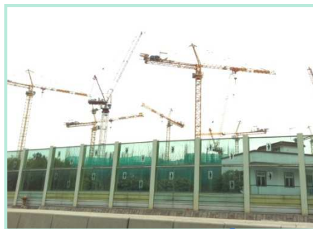
Tai Tong Road project in Feb 2012
