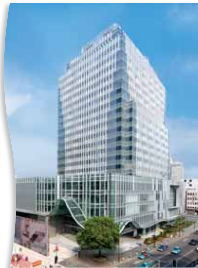
Henderson Metropolitan, Huangpu District, Shanghai
