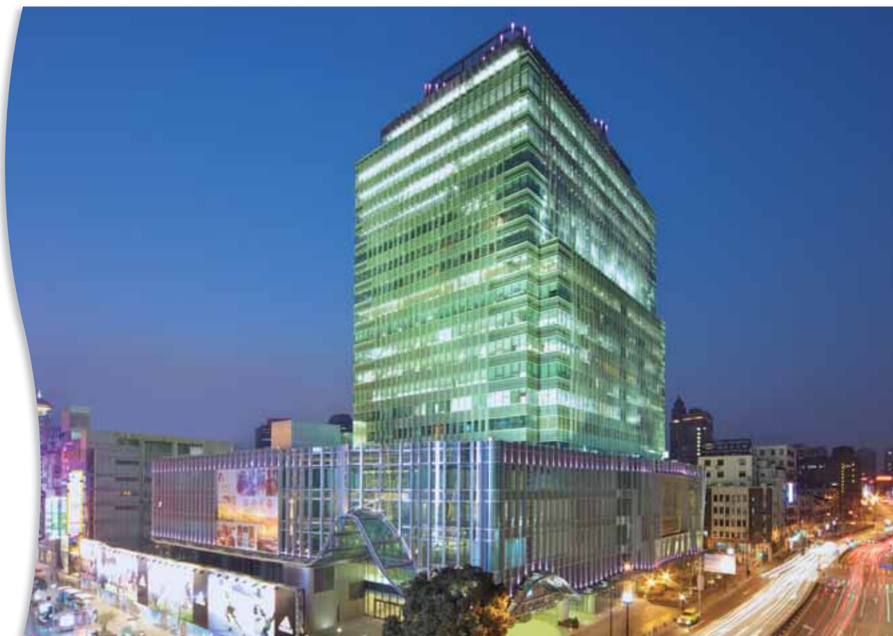
Henderson Metropolitan, Huangpu District, Shanghai
