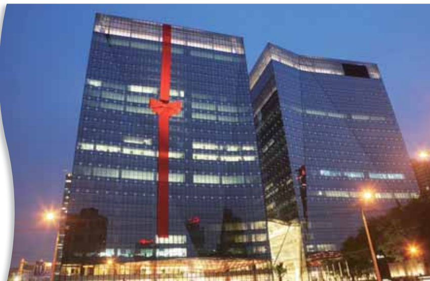
A giant red ribbon was tied around the East Tower of World Financial Centre Beijing to mark its grand opening.
