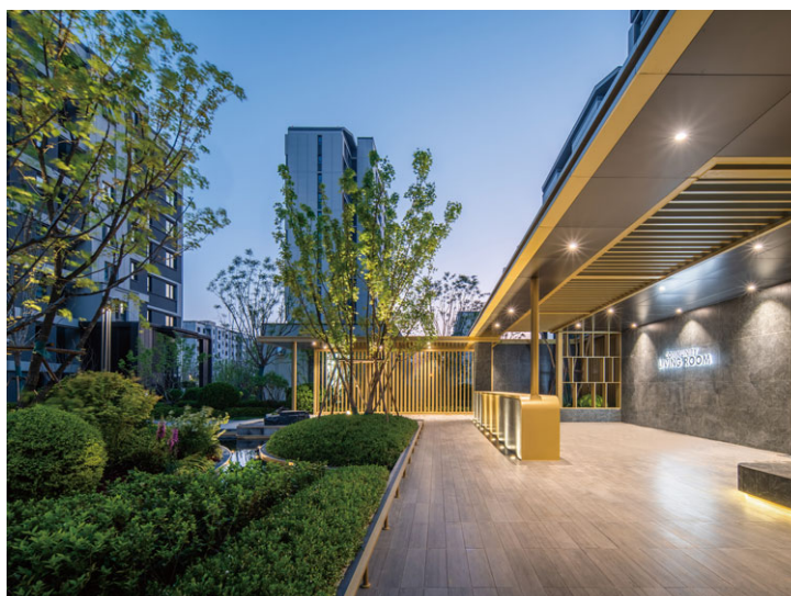
Dongli Project, Tianjin
