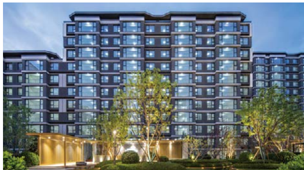
Dongli Project, Tianjin
