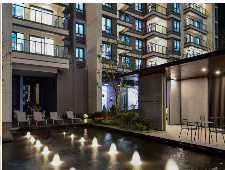
Yubei Project, Chongqing
