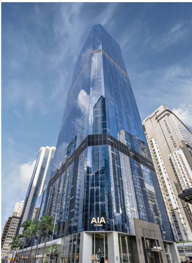
AIA Tower, North Point, Hong Kong
