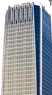
Lumina Shanghai Phase 1
